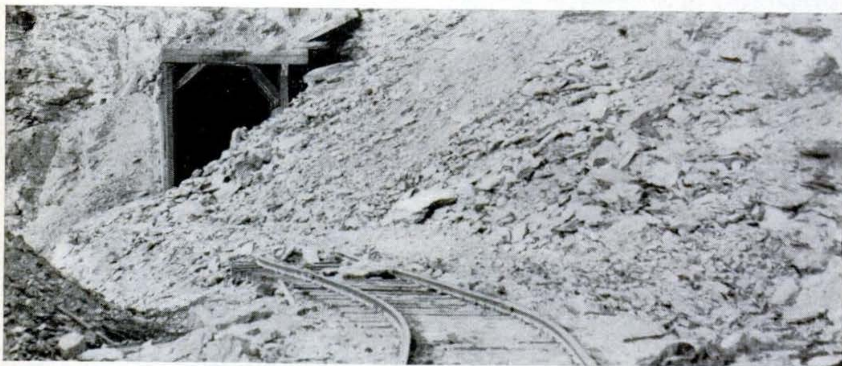
A ROCK SLIDE in the area of the moving mountain blocks 165 feet of track. To prevent another such slide, Army bazooka teams blasted
